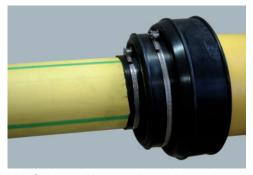
4. Wrap the annular space with the conical part of the S-shaped sleeve and attach it to the carrier pipe with the second strap.
