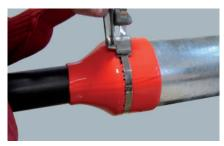
3. When reaching maximum stress, slowly bend over the strap about half a turn while releasing the crank.
