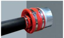
**5.** Inject the adhesive underneath the sleeve the way you did with the casing pipe side and install the second strap. Spread leaking adhesive, if necessary.
