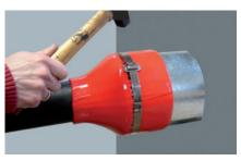
**2.** Install the first strap about 15mm in front of the end of the casing pipe.
