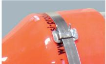
1. Push the stainless steel loop onto the strap; make sure that the barbs point to the end of the strap. Bend over the end of the strap about 3 to 4 cm and strike it with a hammer. Then place the strap around the sleeve and pull it through the loop.
