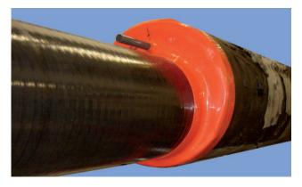
Pull casing end seal over the pipe and mount steel straps (included in the delivery).
